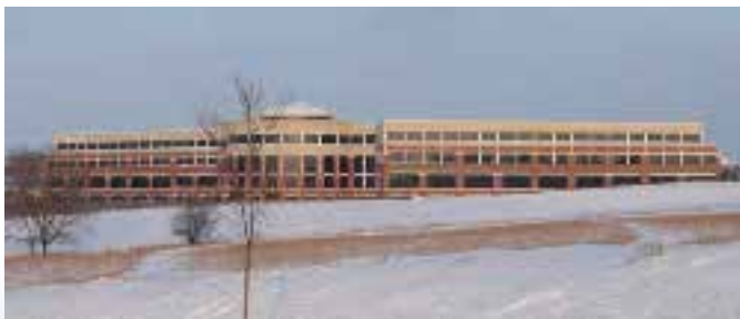
The utilities' head quarters was originally conditioned by seven air handlers utilizing electric steam humidifiers. After deciding to go green, Alliant turned to MeeFog.
