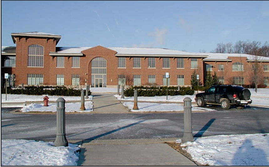
The humidity at NSF International in Ann Arbor, MI, is controlled by an adiabatic humidification system, consisting of a single high-pressure pump. Once the water reaches 1,000 psi, it is distributed to the air handlers.
