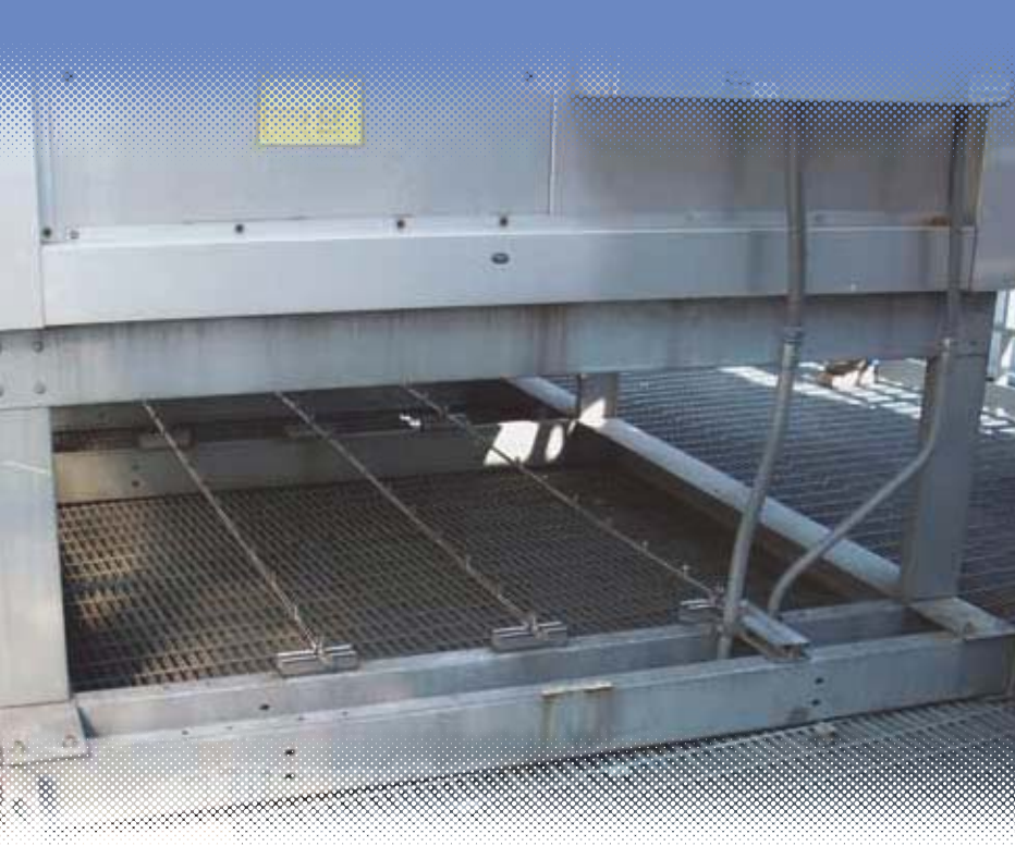
LEFT: Nozzles produce billions of tiny fog droplets that evaporatively cool the inlet air close to the wet bulb temperature.
