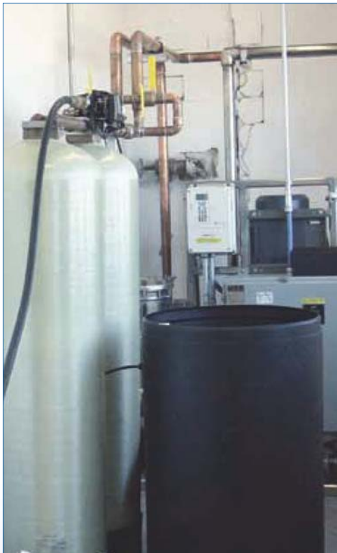
The removal of minerals from the water supply reduces maintenance and prevents fouling of the heat exchanger.
