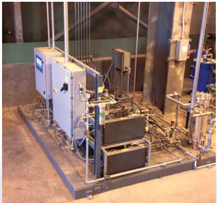
The MeeFog system installed on-site.
