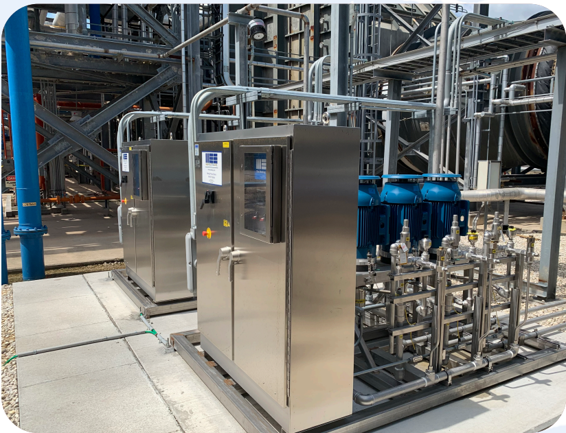
The MeeFog pump skid provides high pressure water to fog manifolds located at turbine inlet.
