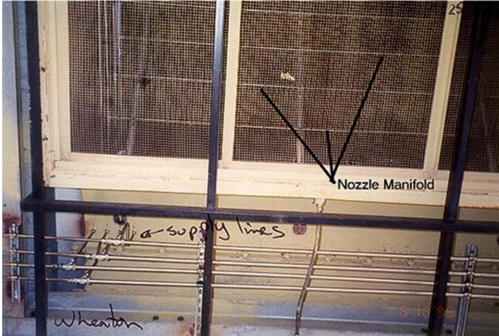
**Figure 11. Nozzle Manifold**
