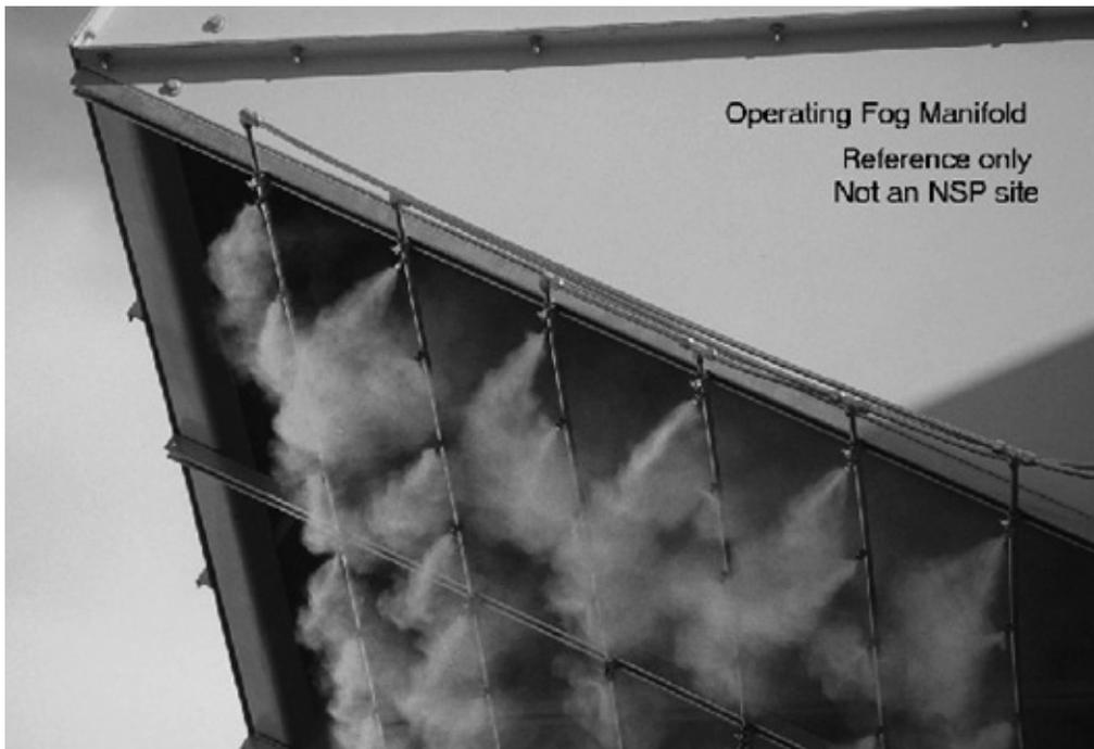
Figure 3. Operating Fogging Nozzle
