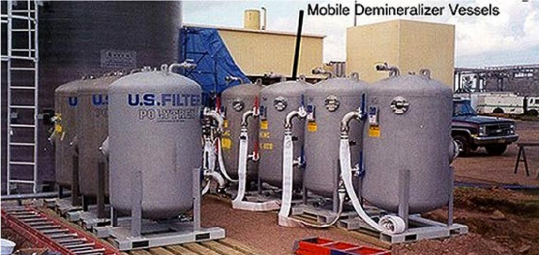
Figure 7. Mobile Demineralizer Vessels
