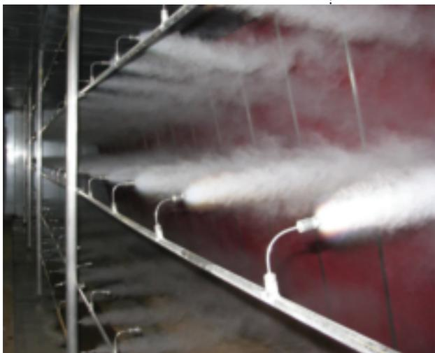
**Fog manifolds run independently to stage the amount of humidification supplied.**
