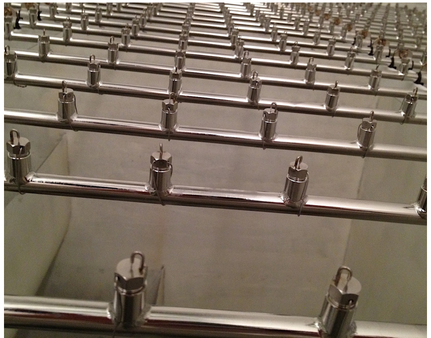
MeeFog Nozzle Manifolds
