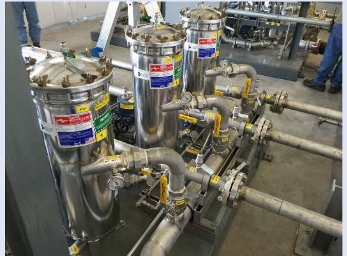
Self-contained MeeFog pump skids are pre-engineered and can be quickly modified for specific applications.
