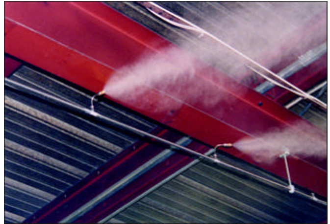
Figure 2 ~ SwirlJet Nozzles
