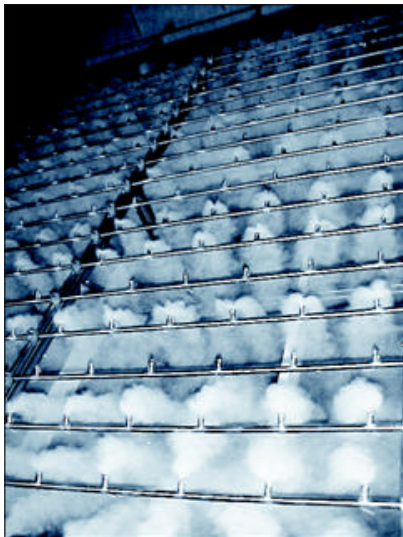
Figure 3 – MeeFog Nozzle Manifold
