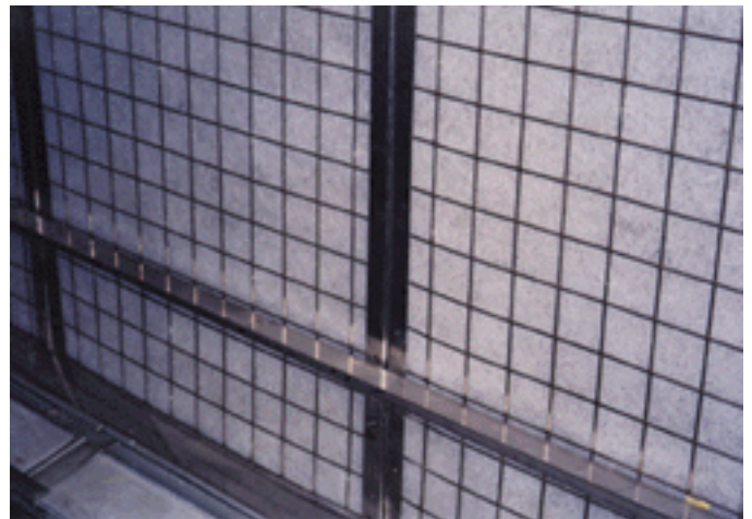
Figure 5 – MeeFog Droplet Filters
