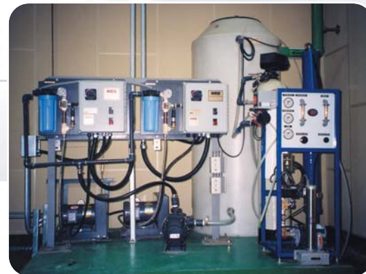
Proven Mee Fog system pumps are conservatively designed to operate below 70% of rated output which translates into high field reliability and service life.
