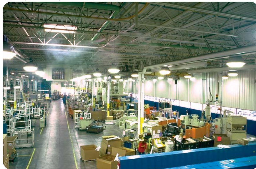
Plant humidification with a Mee Fog system.
